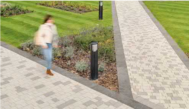
✓ Stretcher-bond paving perpendicular to direction of travel on footways, carriageways
