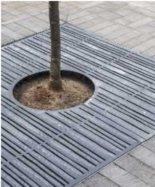
✓ Tree grilles aligning with paving and utilising below-ground wires and guys
