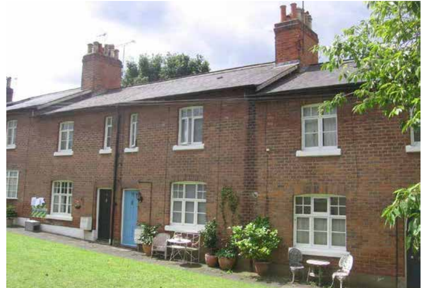
Figure 4.8 Typical houses in the Railway Terraces Conservation Area
