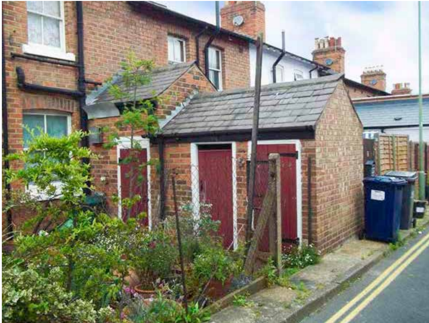
Figure 4.5 Photograph of a typical rear elevation in the Railway Terraces Conservation Area
