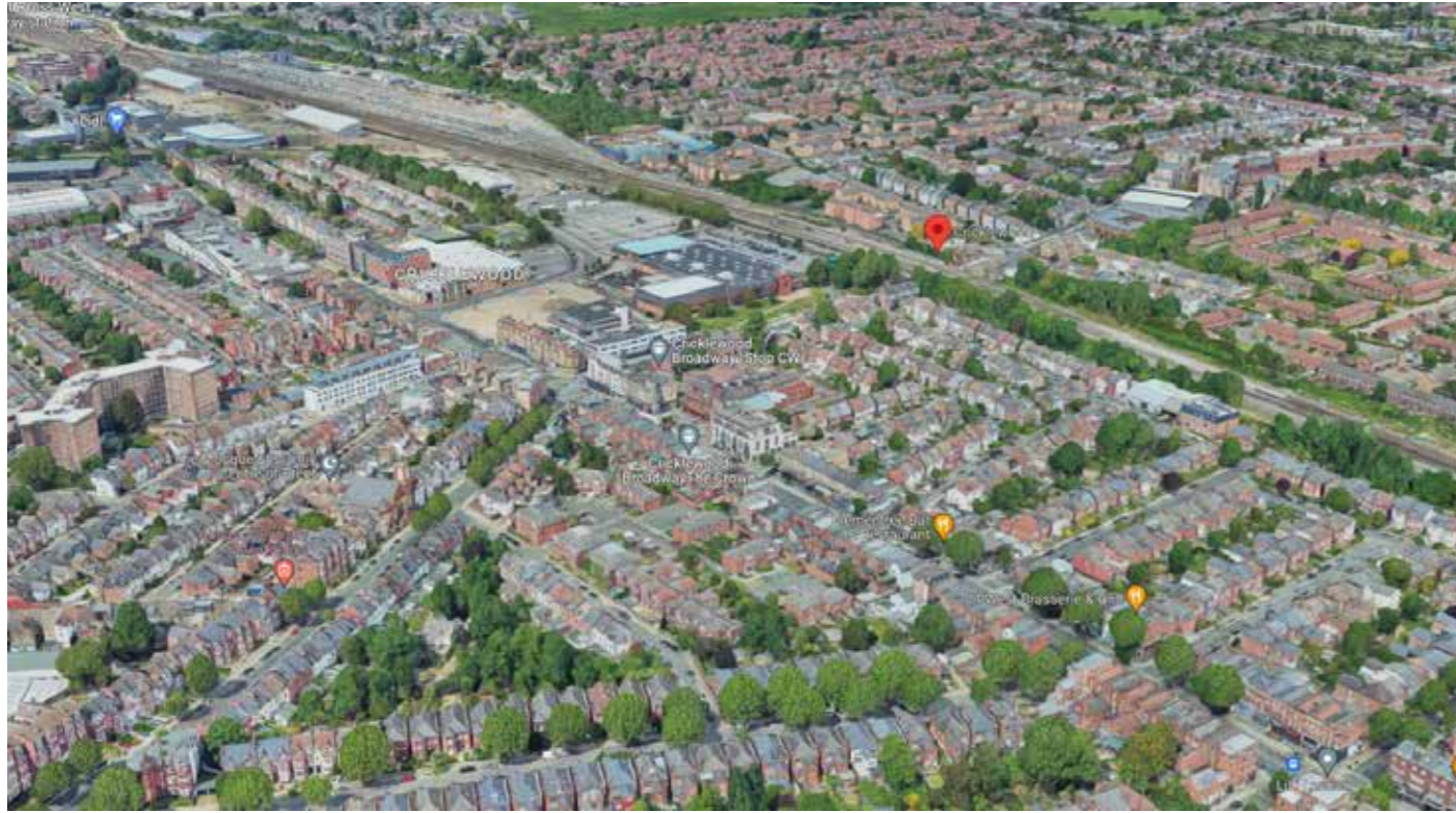
Figure 4.9 Oblique aerial showing wider context
