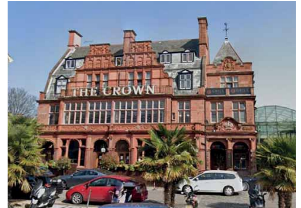
Figure 5.15 The Crown Public House as viewed from Cricklewood Broadway
