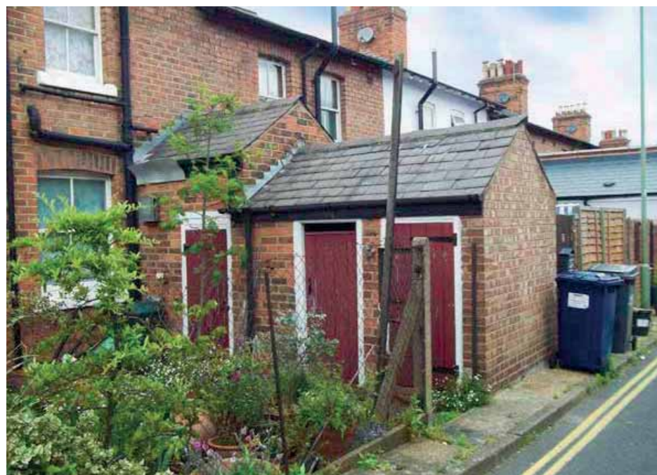
Figure 5.5 Typical rear elevation within the RTCA with outdoor toilet and coal store
