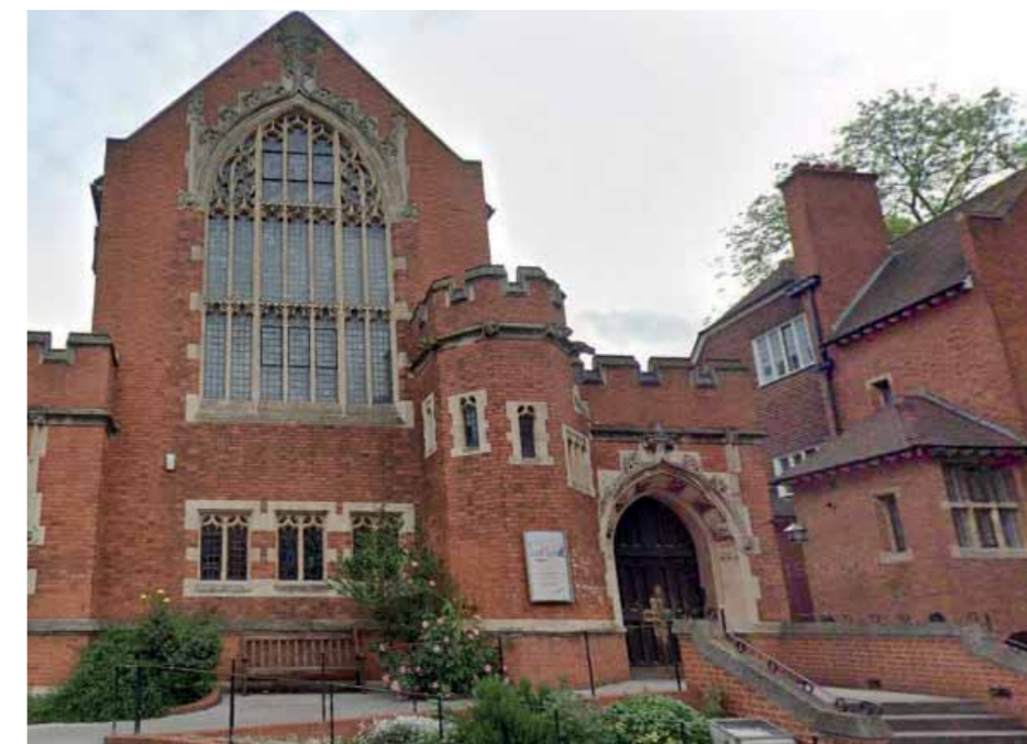
Figure 5.13 Principal south elevation of St Luke’s Church viewed from Kidderpore Avenue
