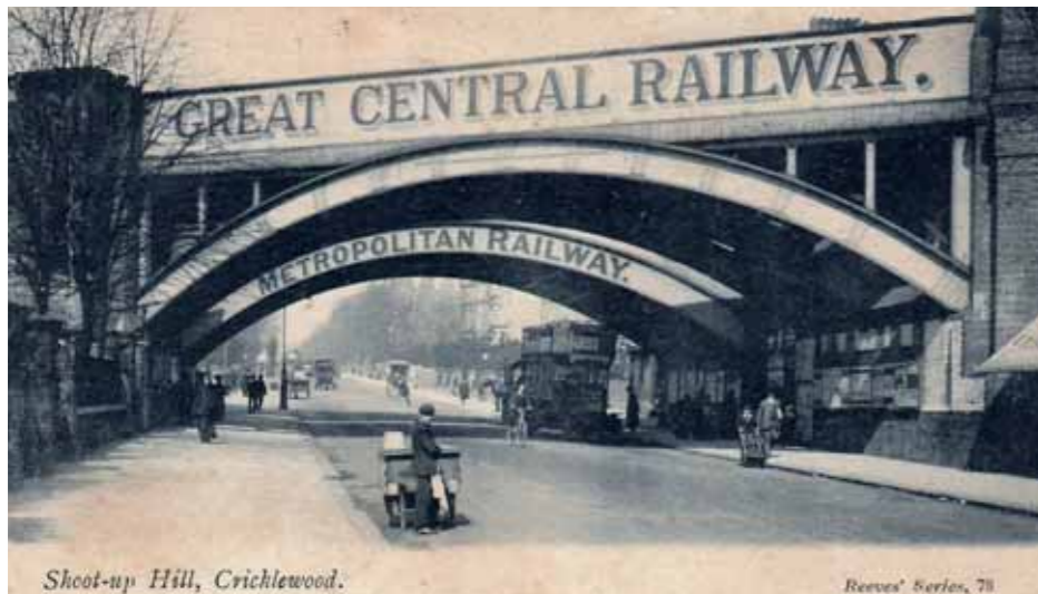
Figure 3.4 The Metropolitan Line Bridge at Shoot-up Hill in the late-C19
