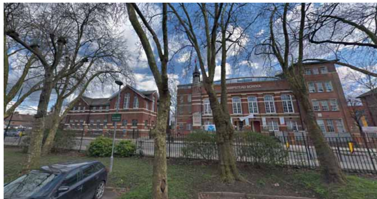
Figure 5.29 The northernmost and central principal buildings at Hampstead School as viewed from the west
