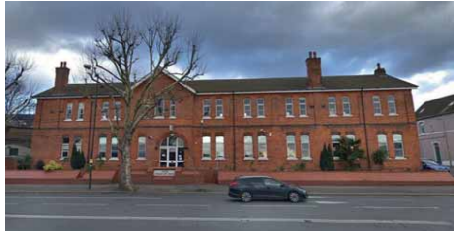
Figure 5.24 The principal west elevation of 318 Cricklewood Broadway
