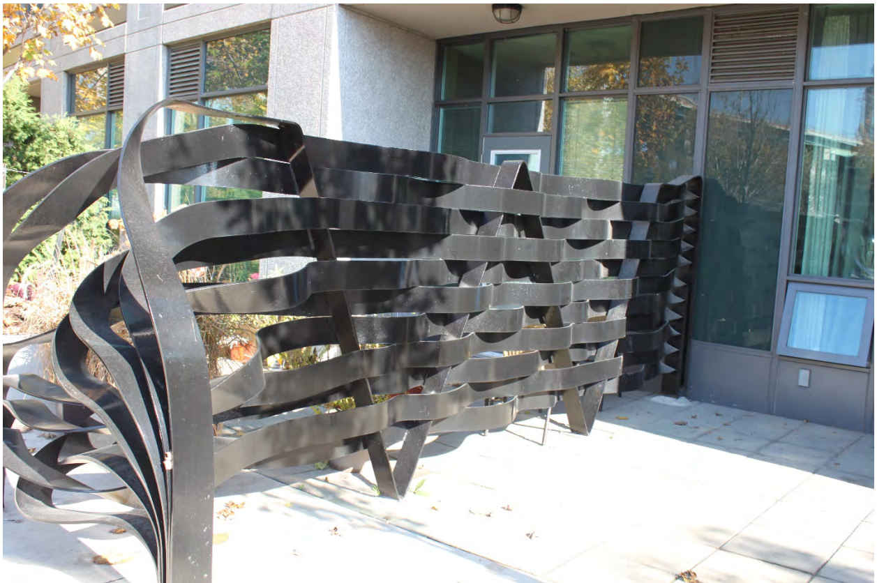
Figure 28: Porous Screen to Mitigate Wind Conditions for Seating Areas
