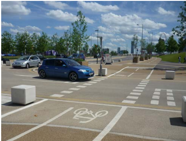
Bent-out cycle tracks with priority at Waterden Road, Hackney. Note that elephants' footprints should not be used to mark this kind of crossing
