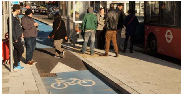
Uncontrolled pedestrian crossing of cycle tracks (at a bus stop bypass)
