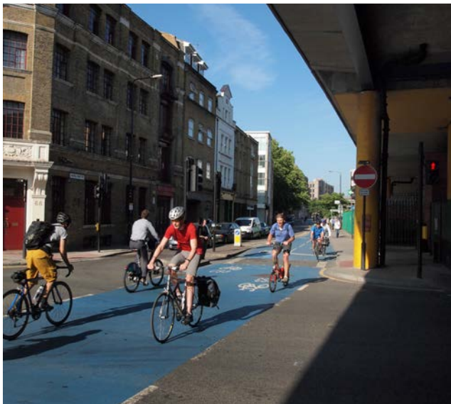
At least 3 metres width is usually needed for comfortable two-way cycling Cable Street, Tower Hamlets
