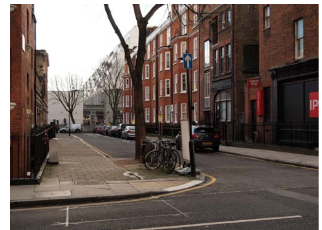
Footway build-out incorporating cycle parking
