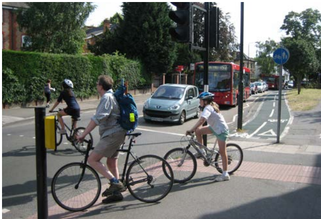
Toucan crossings are often used to carry off-carriageway tracks through or around junctions
