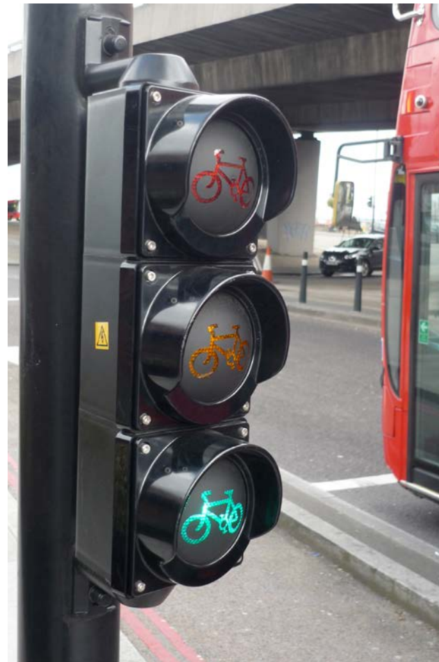
Detail of low-level cycle signal
