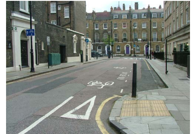
Footway build-out with contraflow cycle provision
