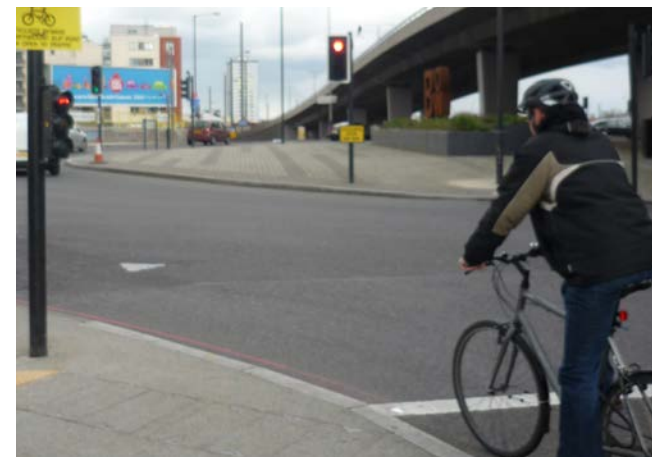
Cycle gate at Bow: (top) segregated approach and first cycle stop line, and (bottom) advanced cycle stop line. Trial low-level cycle signals (used as repeaters) are mounted below the main signal heads
