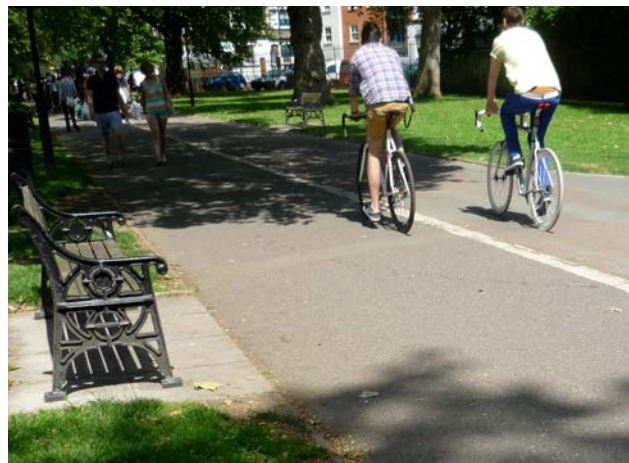
Partial (white line) separation in London Fields
