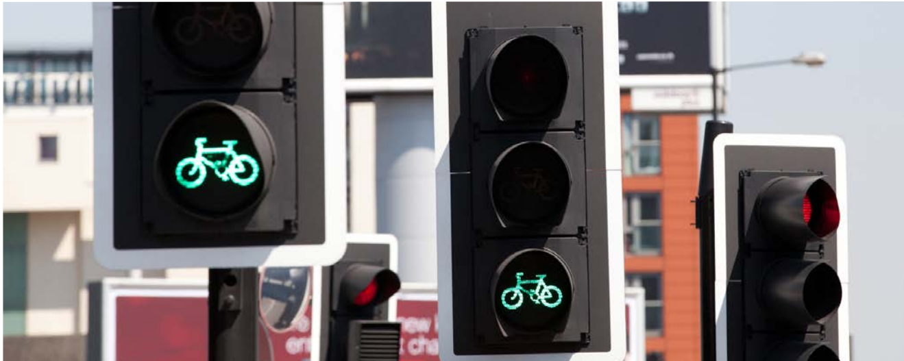
Standard signal heads with green cycle aspects
