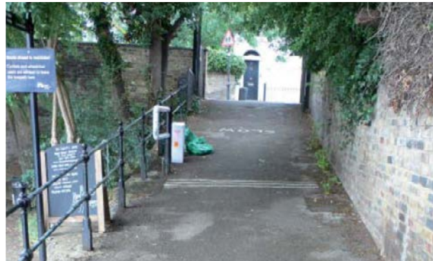
Ramp to Regent's Canal towpath, Danbury Street: use of 'slow' markings and rumble strips to remind cyclists to ride slowly downhill. Well maintained vegetation helps to maximise width and visibility
