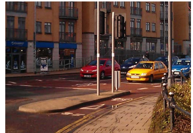
Bypass to traffic signals for left-turning cyclists, Hills Road / Cherry Hinton Road, Cambridge
