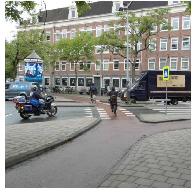
Roundabout with off-carriageway tracks in Amsterdam
