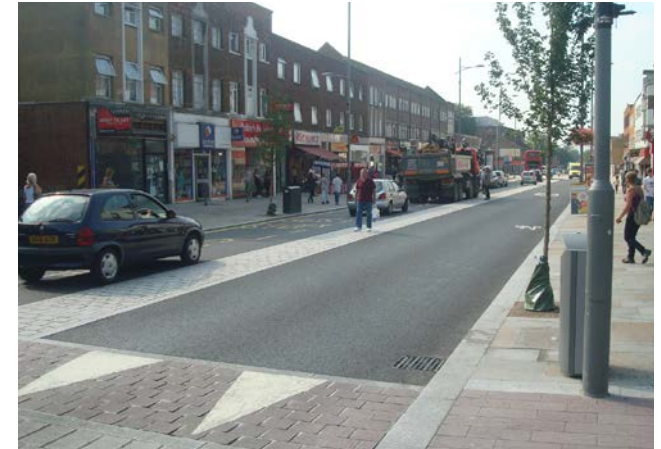
Flush median strip, Bexleyheath
