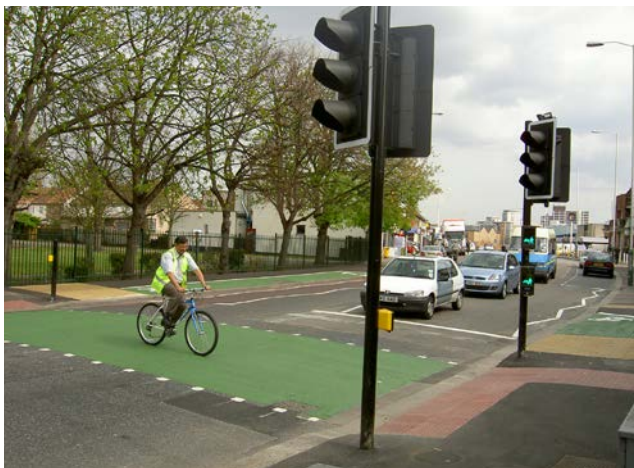
Typical toucan crossing arrangements, with shared use and tracks on either side (colour optional)
