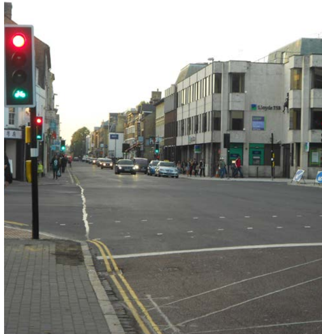
Fourth aspect on standard signal head, giving cycle early release at Hills Road, Cambridge
