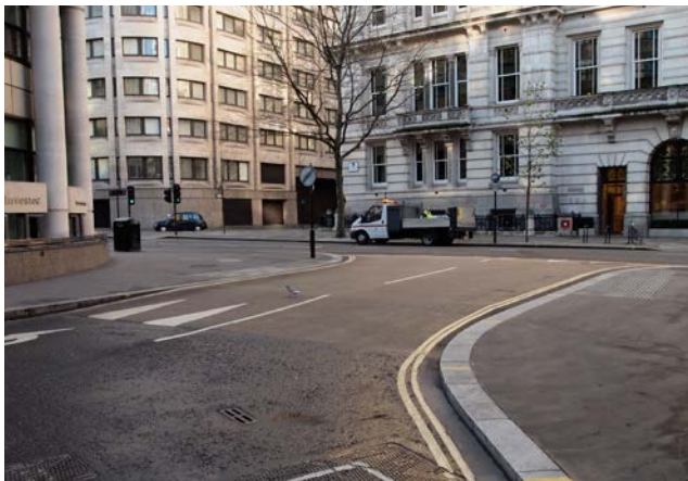
Shallow ramp up to entry treatment, Gresham Street, City of London
