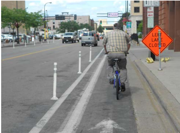
Light segregation with posts in Minneapolis
