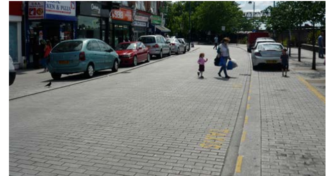
Minimal kerb upstands – Byng Place, Camden and Church Lane, Leytonstone
