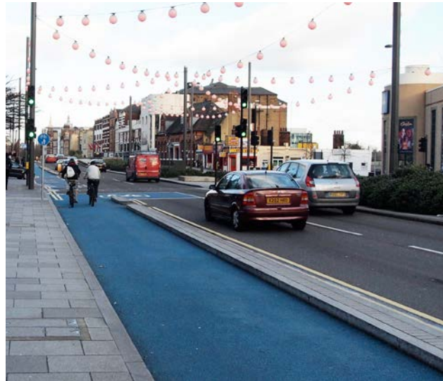
Full segregation on CS2 extension
