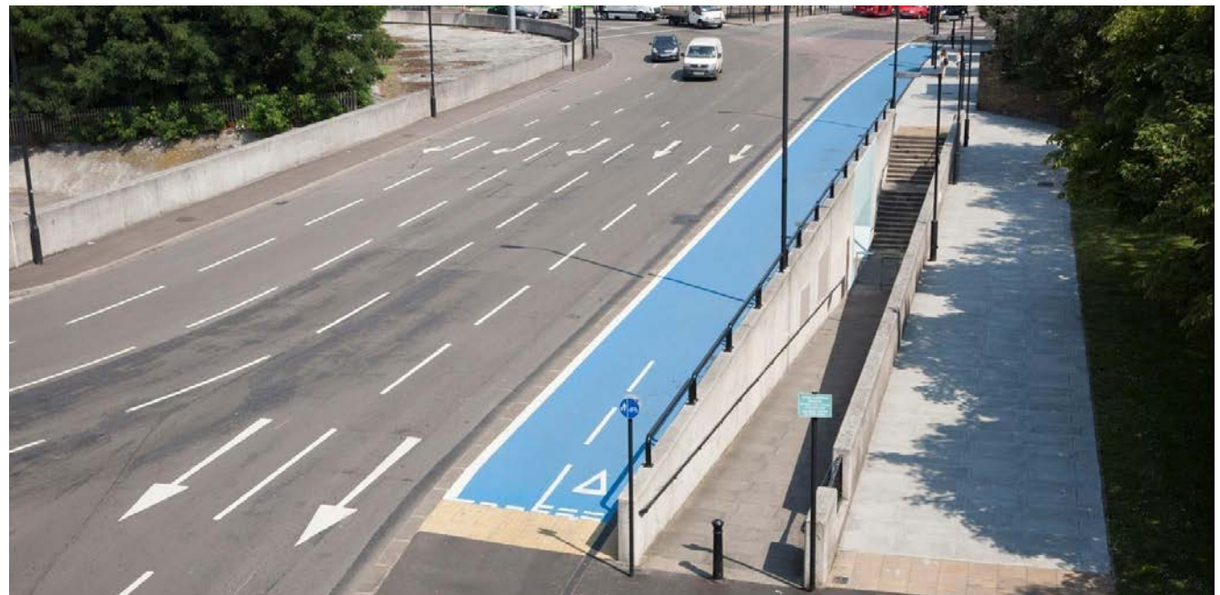
General traffic lane converted to off-carriageway tracks at Wandsworth Gyratory
