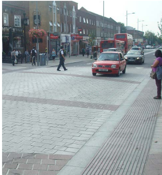
Corduroy paving used instead of a kerb edge at Bexleyheath
