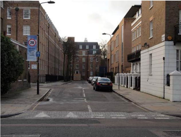
Entry treatment with asphalt table, Gray's Inn Road/Heathcote Street, Camden
