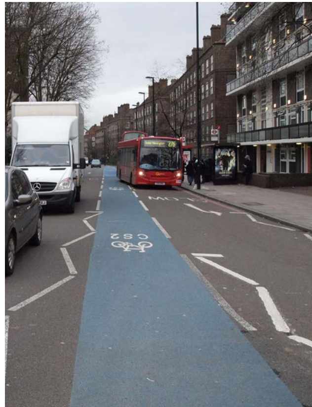
Long central lead-in to allow for left-turn flare, positioned to facilitate overtaking stopped buses
