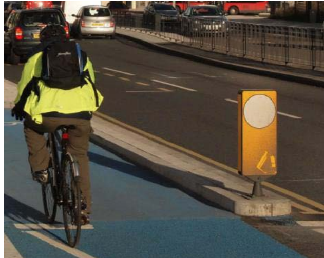
Blank bollard (without recommended clearance)
