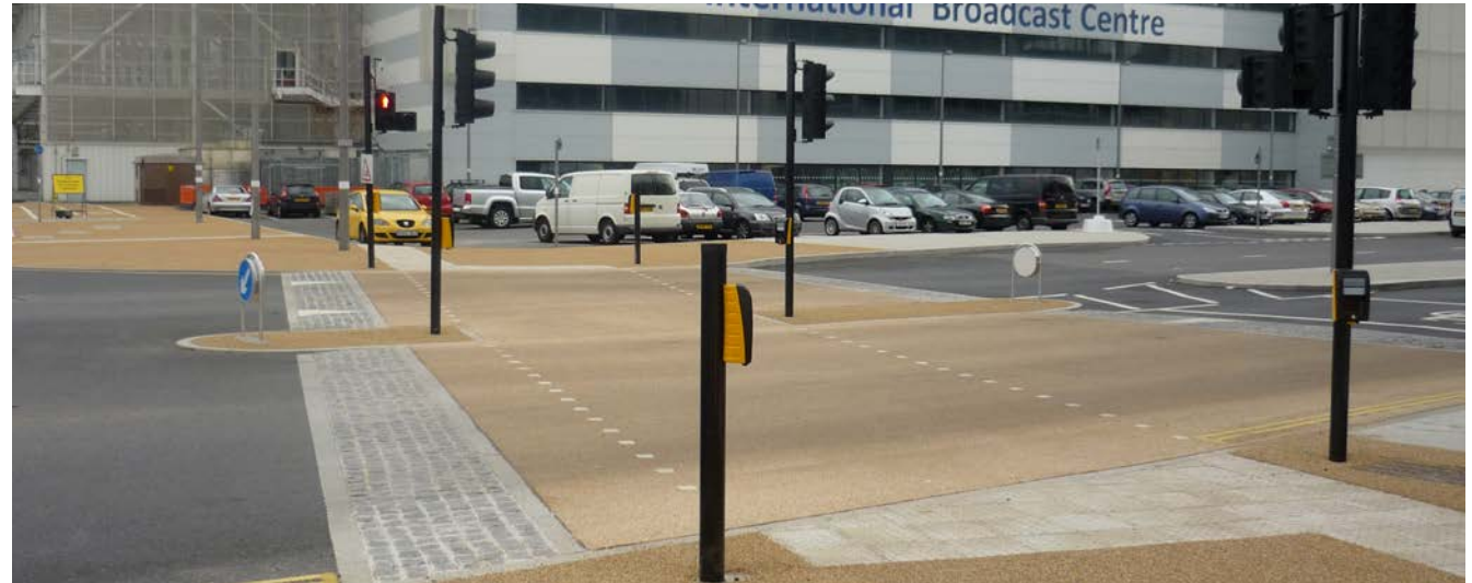
Crossing on a raised table and with contrasting surface treatment, Waterden Road, Hackney
