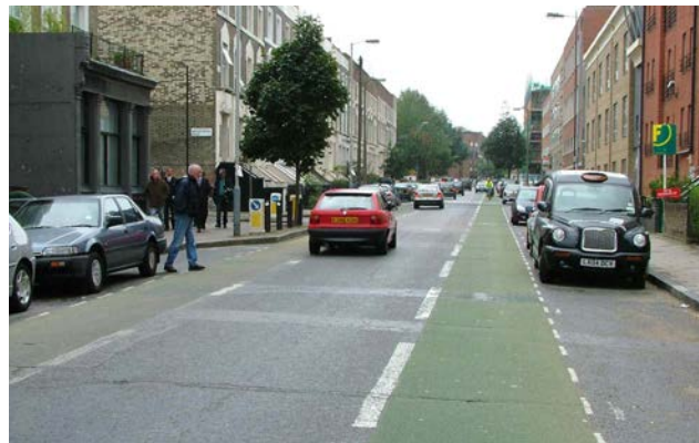
Advisory lanes on two-way streets with no centre-line – wide (left) or buffered (right) to account for parked cars
