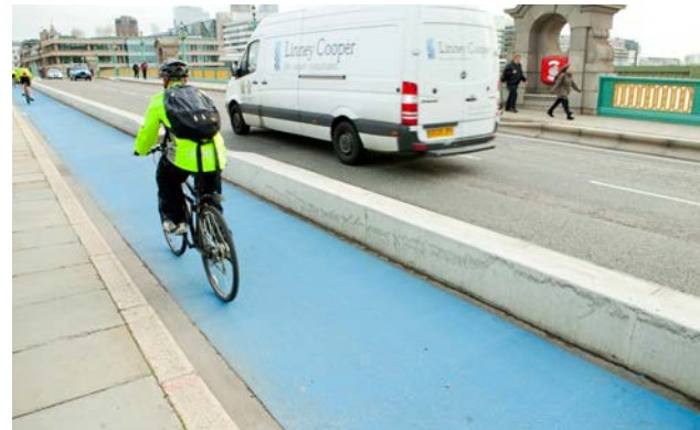
Kerbed separation, Southwark Bridge
