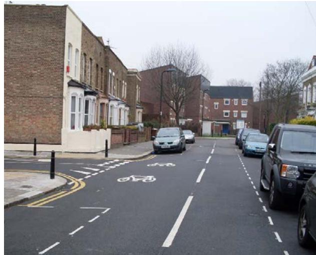
TSRGD diagram 1057 symbols positioned so as to mark a cycle route through a junction
