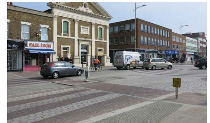
Informal roundabouts at Moor Lane, City of London and Bexleyheath town centre, both of which have a ‘roundabout-like’ feature in the carriageway
