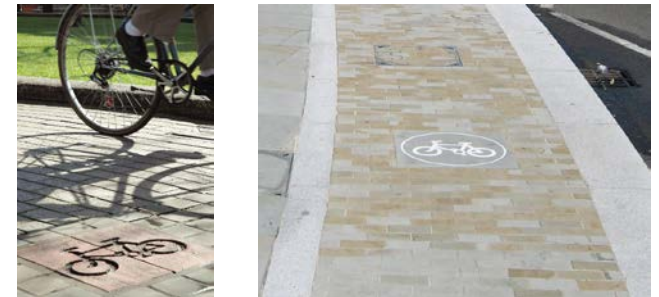
Non-prescribed uses of the cycle symbol, to show that cycling is permitted
