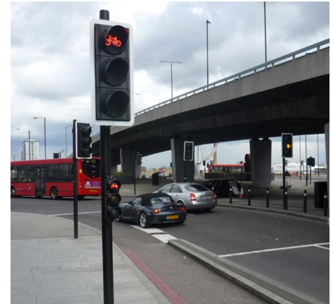
High-level red cycle aspect with low-level cycle signal used as repeater
