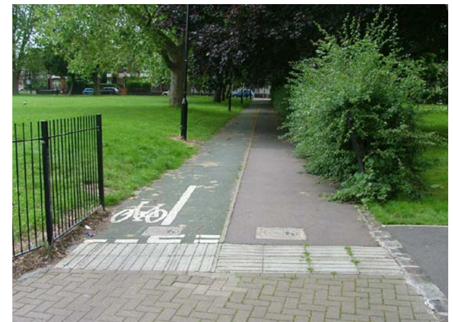
Separation using colour, symbols and tactile paving (note that regulatory 'give way' markings should not be used here)
