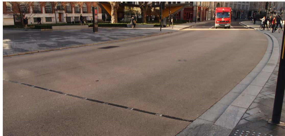
Wide crossing, consisting of two parallel stand-alone, signal-controlled crossings, with contrasting surface treatment, St Paul's Churchyard, City of London
