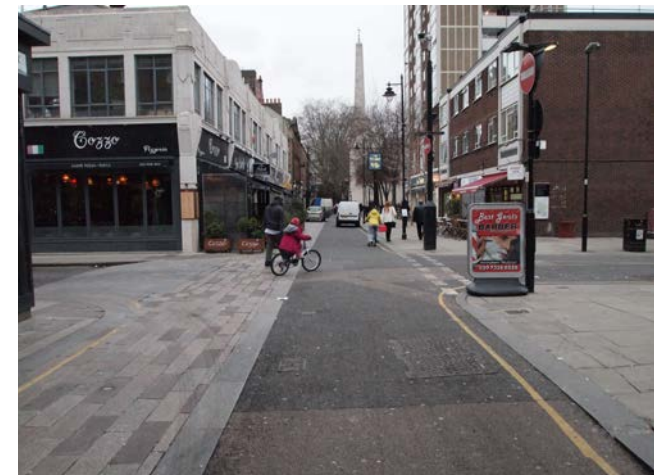
Visual narrowing of the carriageway at Whitecross Street, Islington. Stalls are set out on the paved area when the market is on.
