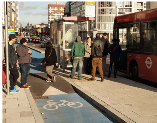
Bus stop bypass at Stratford High Street, showing pedestrian crossing over cycle track
