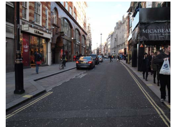
Fully inset loading bays to support retail premises – Long Acre, Covent Garden
