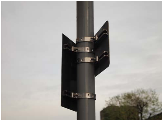
Signs with fixing channels and mounting clips
