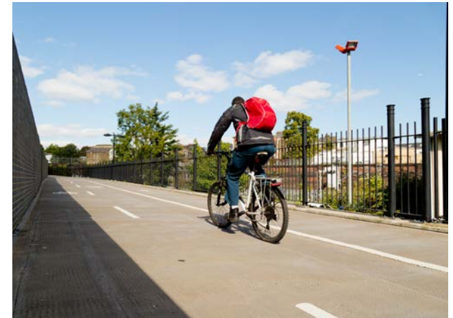
White line separation, with centre lines on cycle track – Camley Street, Camden
