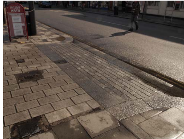
Block-paved entry treatment with tight corner radii – Walworth Road, Southwark
