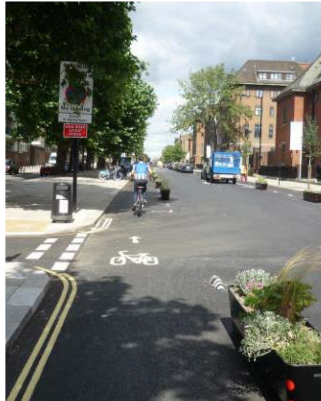
Flexibility of infrastructure at Royal College Street, Camden has allowed for adjustment of lane widths and relatively easy replacement of damaged separators and planters
