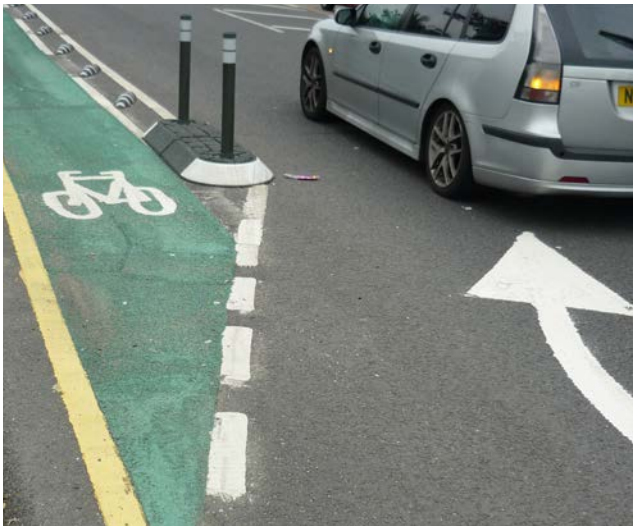
Temporary island at the beginning of a run of separators (Salford trial)
