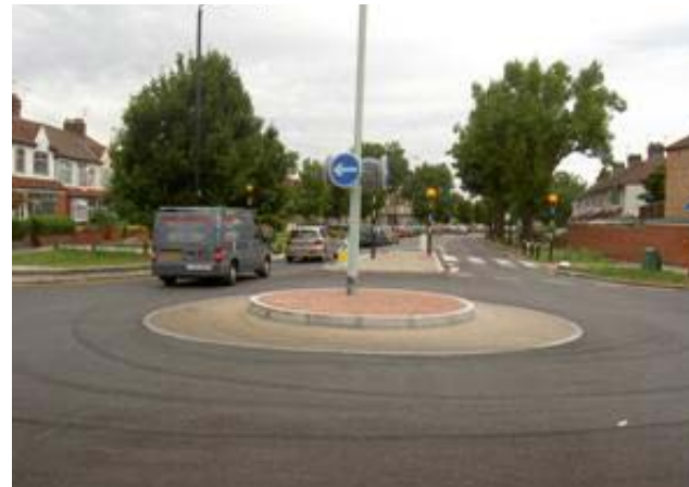
Compact roundabout in UK with overrun strip
