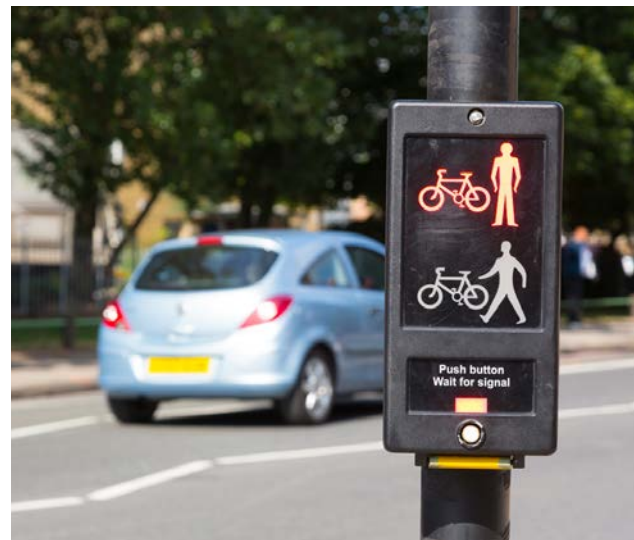
Nearside push-button control for toucan crossing
