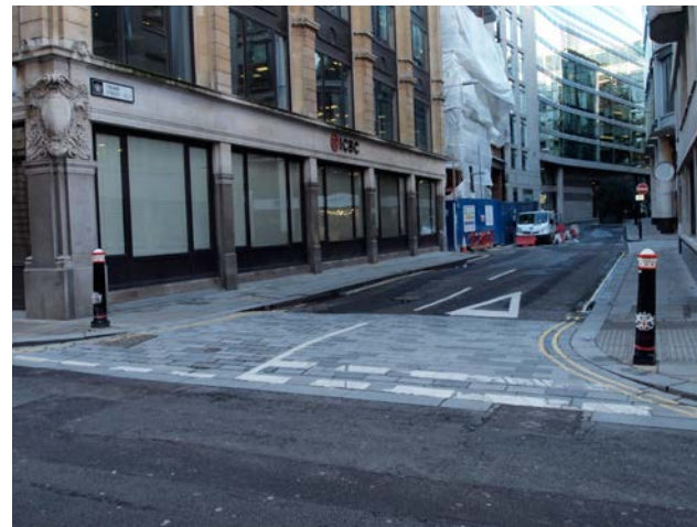
Typical entry treatments in the City of London, with visual contrast with carriageway: at a narrow street with cycle contraflow (Cloak Lane, left) and at a two-way street (Trump Street, right)
