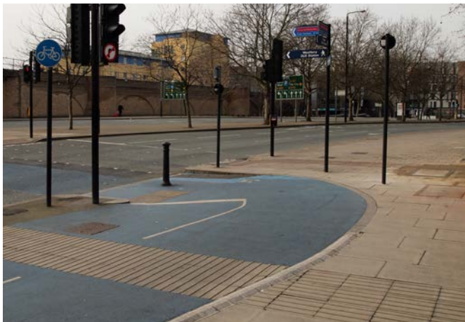
Type [1]: parallel crossings at Westferry and West India Dock Road. Ladder and tramline tactile paving are used for transition from track to shared area
