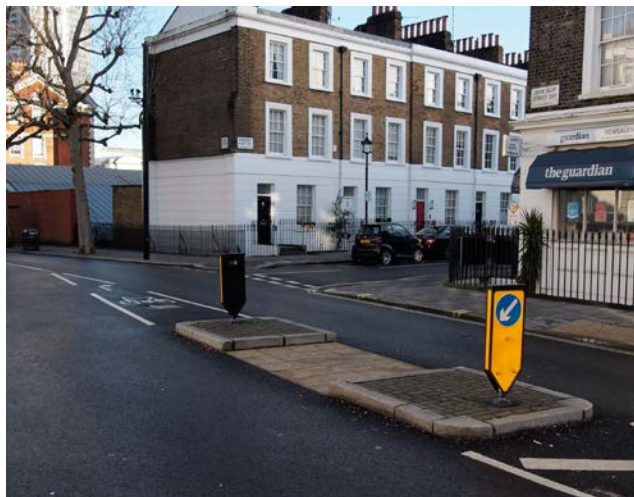
Pedestrian refuge island assists cycle right turn
