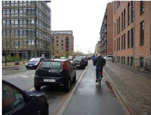
Stepped cycle tracks in Copenhagen (left) and Stockholm (right)
