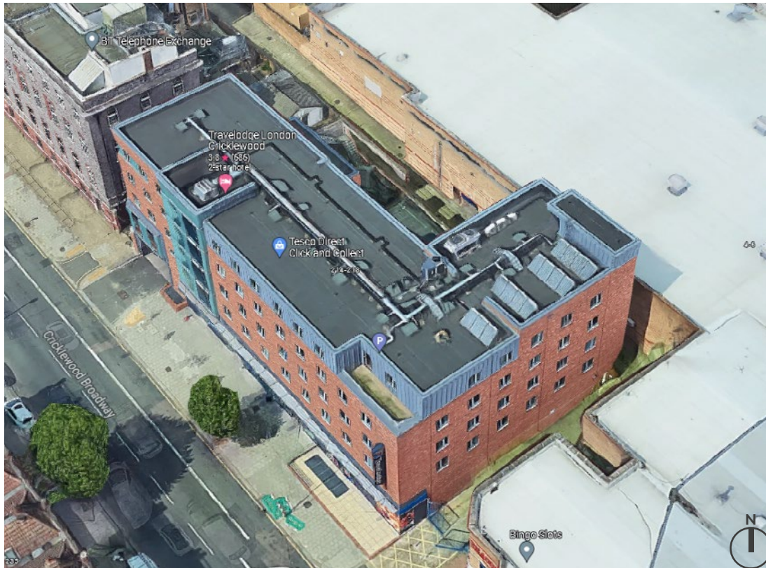
Fig. 16: Existing PV Panels - Aerial view
