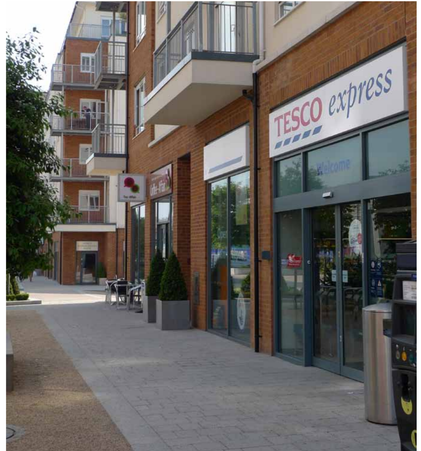
Active ground floor uses help to integrate a taller buildings with the public realm
