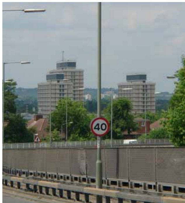
5 - Metropolitan Police Centre, Hendon
