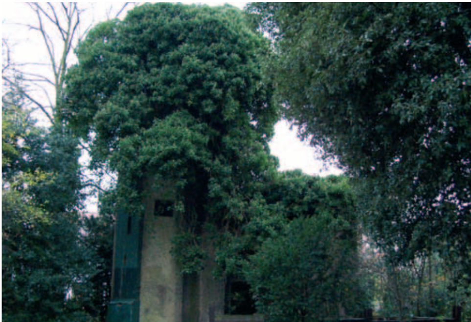
The Water Tower, grade II listed structure at the Avenue House Estate
