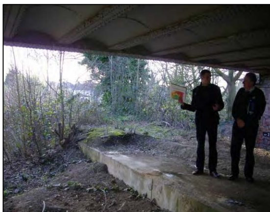
Figure 9 - The Aerodrome Ditch, culverted section under railway
