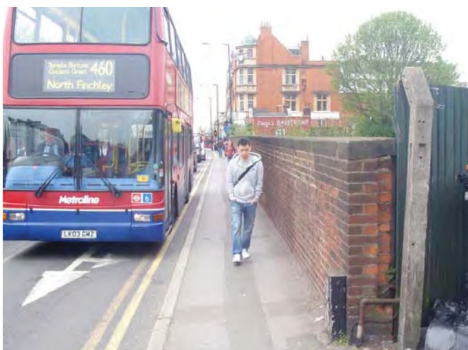
The bridge over the railway lines
