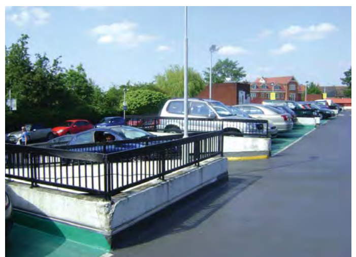
Tesco multi-storey car park
