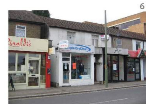
Low quality buildings along East Barnet Road
