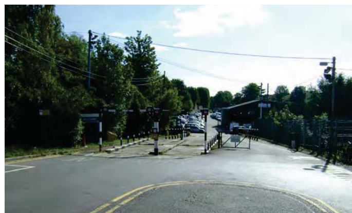
Opportunity site - Finchley Central Station (car parking reprovided)
