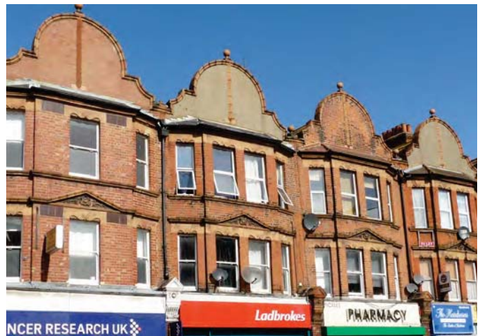
Upper level to historic terraces - Ballards Lane
