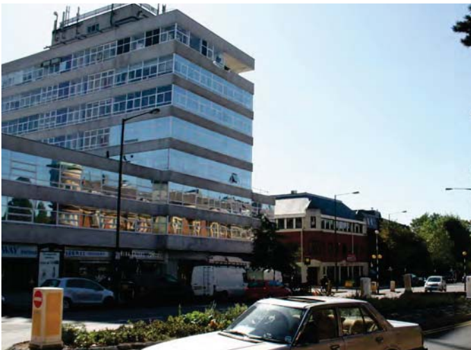
Area 3 - Regents Park Road north (Gateway House)
