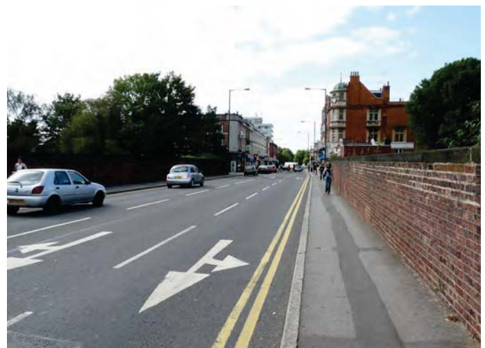
Area 2 - Railway bridge south of Ballards Ln/Nether St junction
