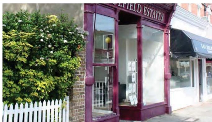
Protect historic shopfronts - Hendon Lane
