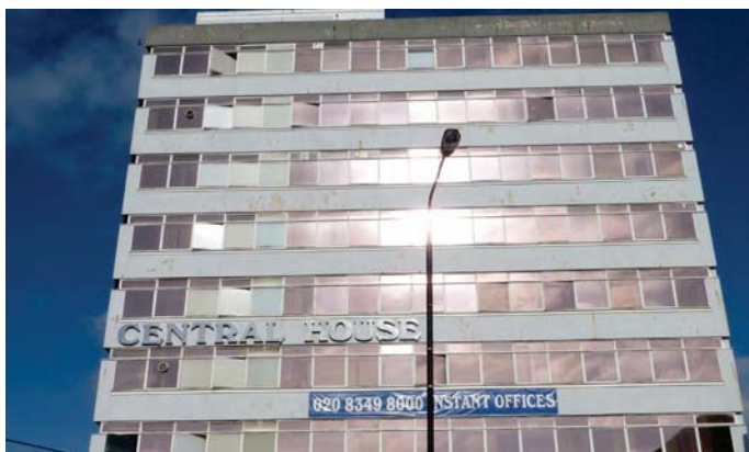
Opportunity site - Central House
