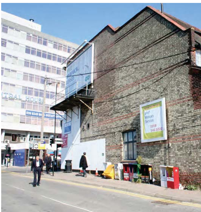
Street clutter, signage and advertising hoardings - Chaville Way
