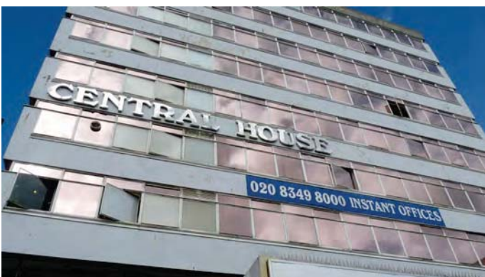
Refurbish or redevelop office accommodation - Central House
