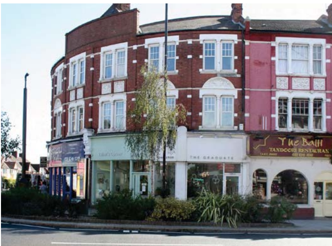
Area 1 - Ballards Lane north
