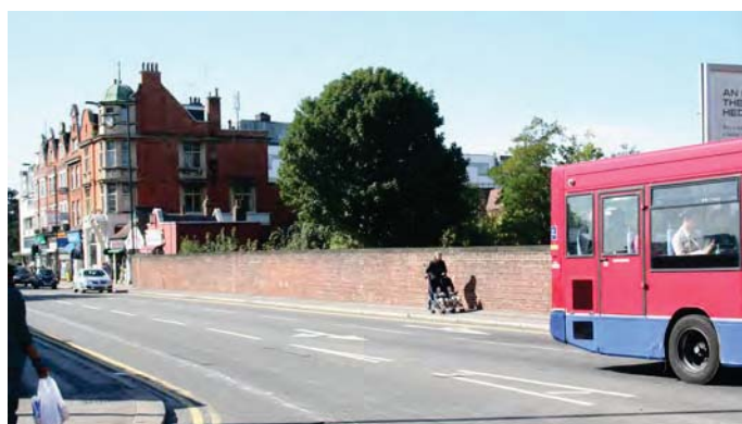
Improve pedestrian accessibility - railway bridge
