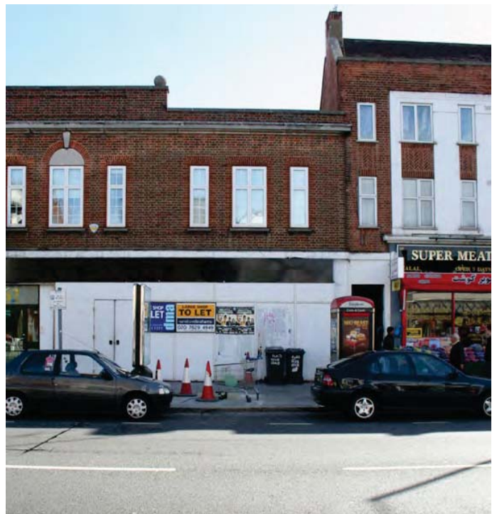
Street clutter and informal signage - Ballards Lane
