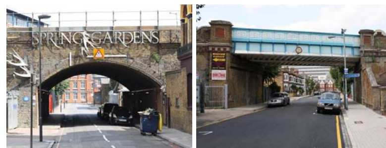
Example of aesthetic enhancements to rail bridges which create a focal point of interest
