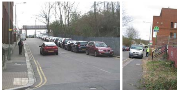
Boundary treatments in New Barnet which need to be improved and maintained
