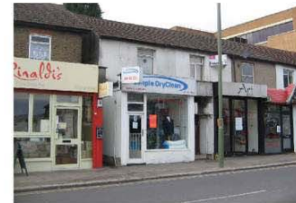
Low quality buildings along East Barnet Road
