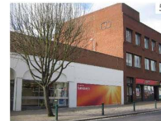
Sainsbury's building has a long continuous frontage along the High Street - white arches out of keeping with built form
