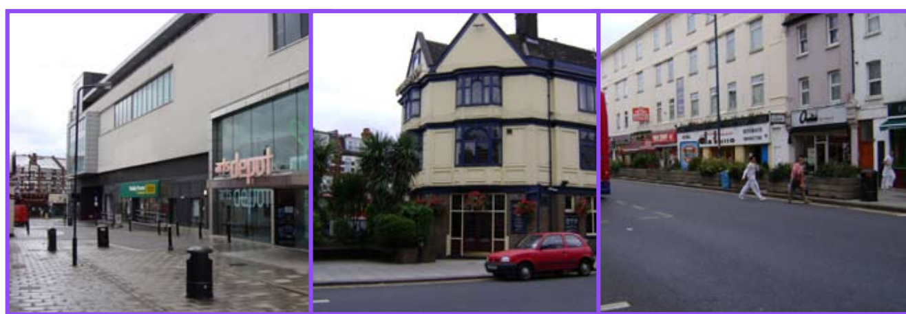
Arts Depot Tally Ho pub Balfour House with restaurants
