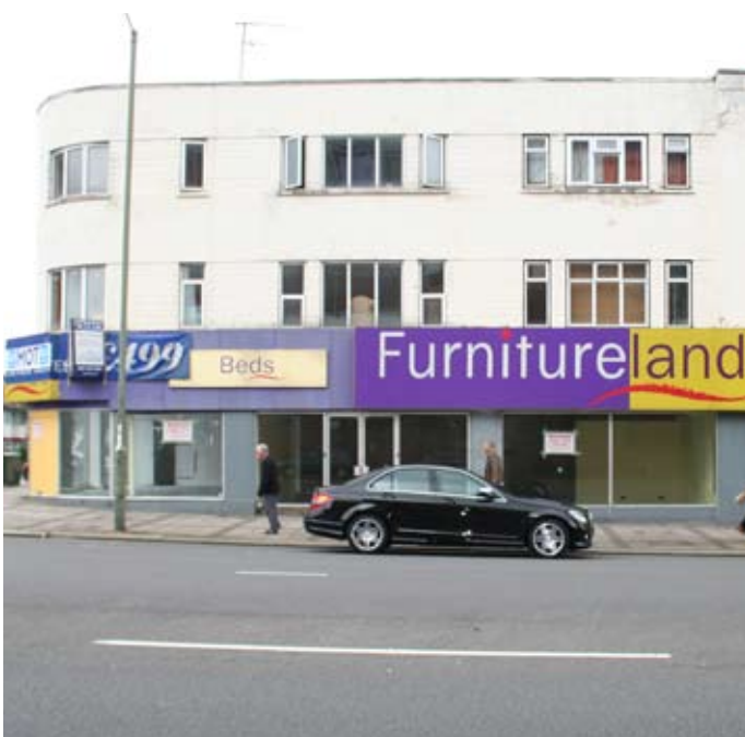
Large vacant retail unit within the Northern character zone
