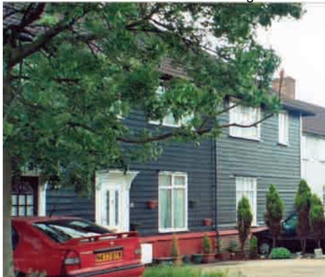
Black stained timber weatherboarding
