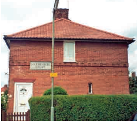
Decorative string course at first floor level
