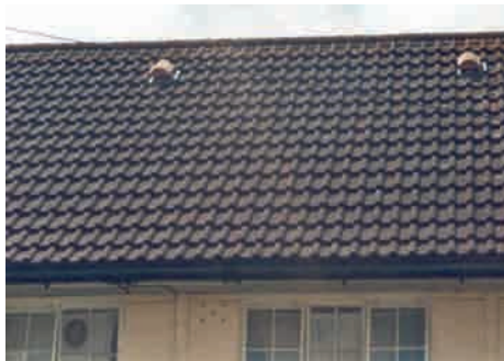
Single roll clay pantiles
