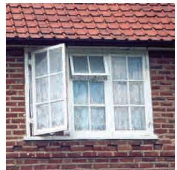
White painted timber casements
